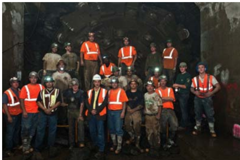
The crew stands before the T.B.M.'s point of entry. Photos courtesy M.T.A.
