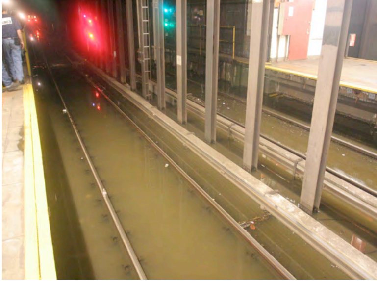
Figure 3 F Line Hillside Ave Related Flooding
