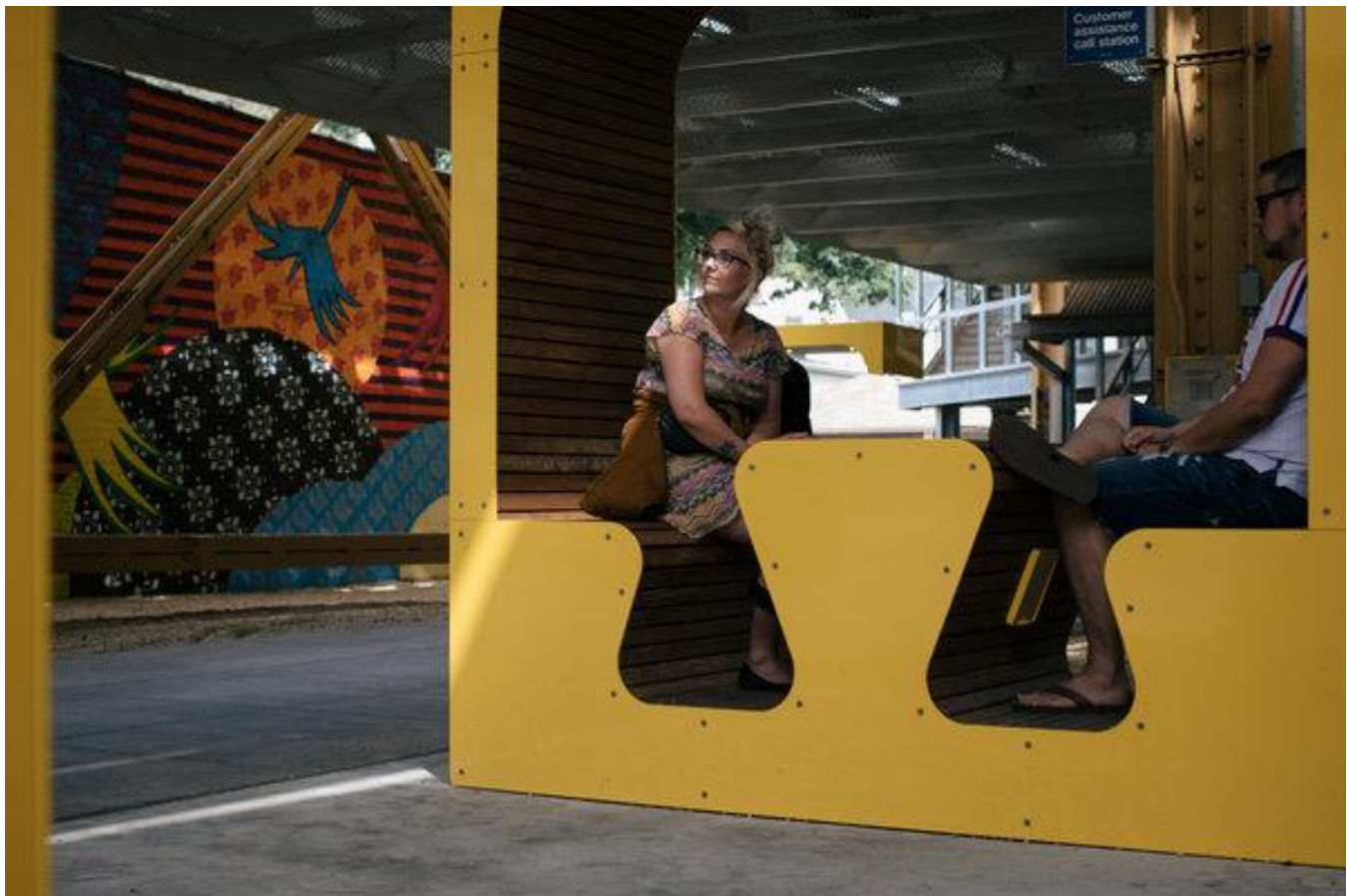
A desolate alley below the elevated tracks of the Paulina Station was converted into a hip plaza with murals and seats. Alyssa Schukar for The New York Times
