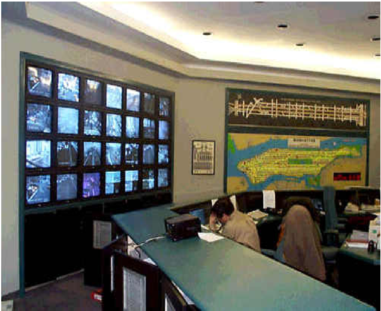
Figure-10 NYC TMC Engineer Monitoring Key Locations
