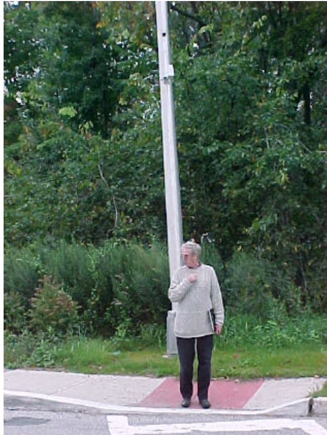
Figure 11. One of the four microwave detectors used to activate the in-pavement flashing warning lights. The detector is in the small box on the pole behind and above the pedestrian.
