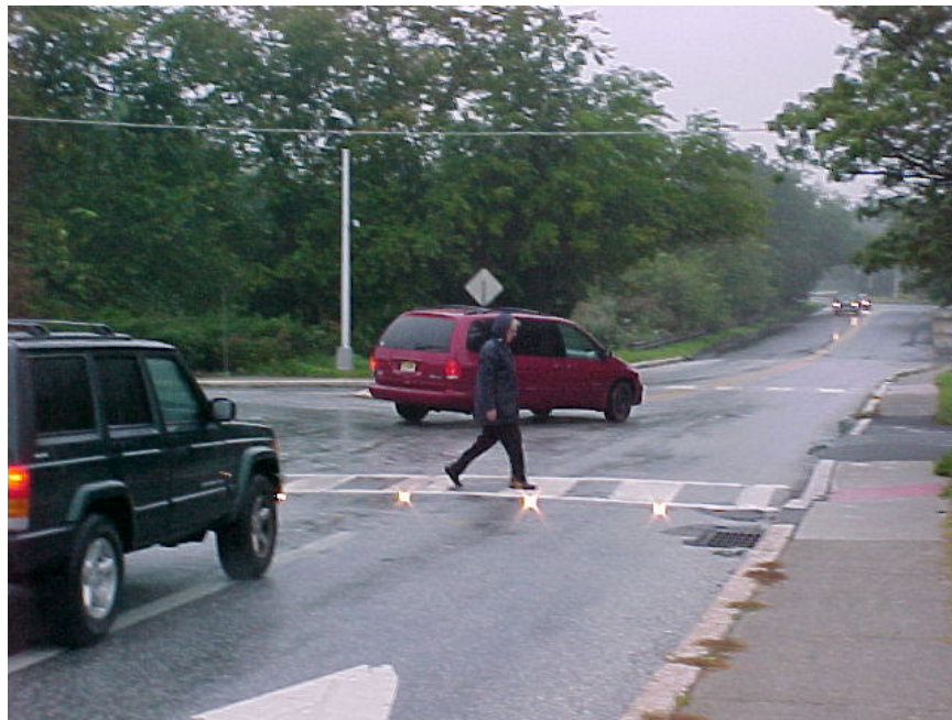
Figure 9. Crosswalk 1 with the in-pavement flashing warning lights installed and operating, at the time of the third evaluation.
