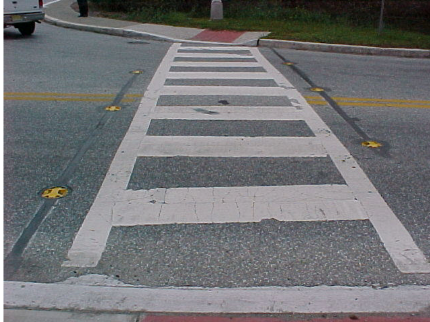
Figure 10. Crosswalk 2 with the in-pavement flashing warning lights installed, at the time of the third evaluation.
