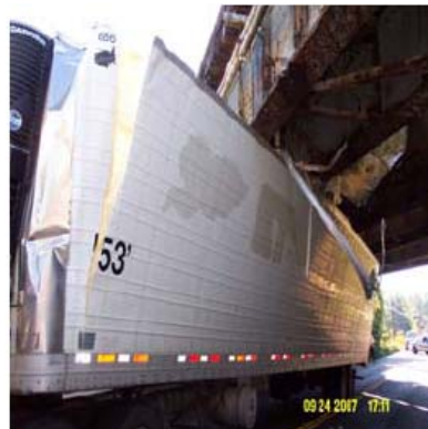
Figure 3-12: Impact to the Bridge 7050634 on Sept. 24, 2007.
