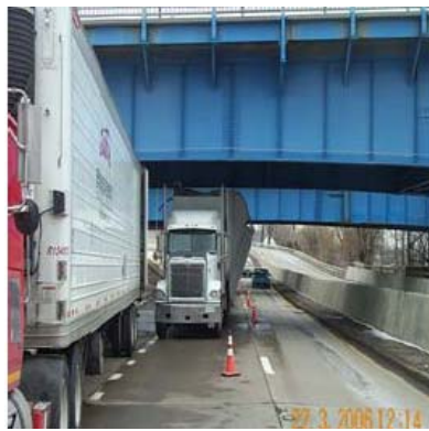
Figure 3-11: Impact to the Bridge 5045751 on March 22, 2006.
