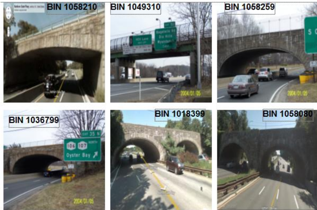
Figure 3-23: Typical Bridges in Region 10 Hit Multiples Times by Trucks.
