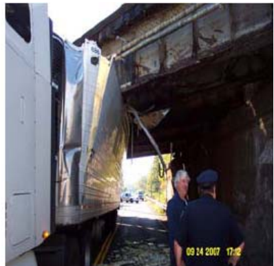
Figure 3-12: Impact to the Bridge 7050634 on Sept. 24, 2007.
