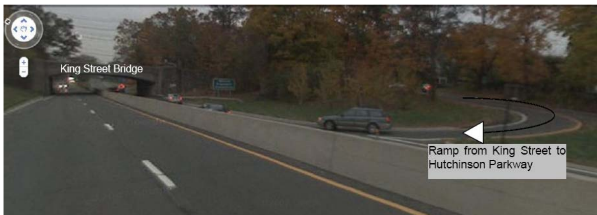
Figure 3-19: Ramp from King Street to Hutchinson Parkway (Photo from Google Maps)
