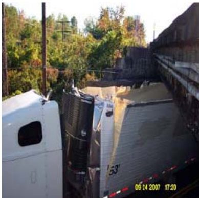
Figure 3-12: Impact to the Bridge 7050634 on Sept. 24, 2007.
