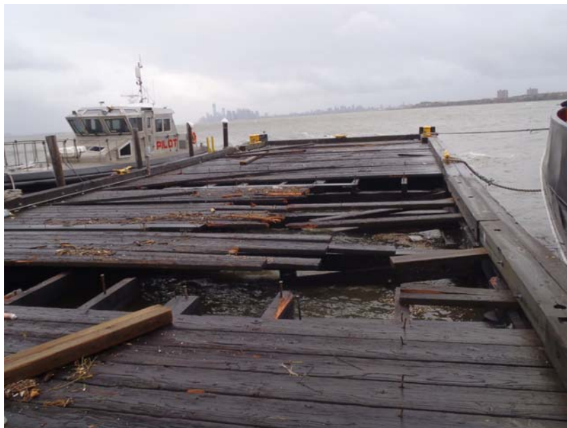
Figure 9: Piers damaged by uplift forces during Sandy
