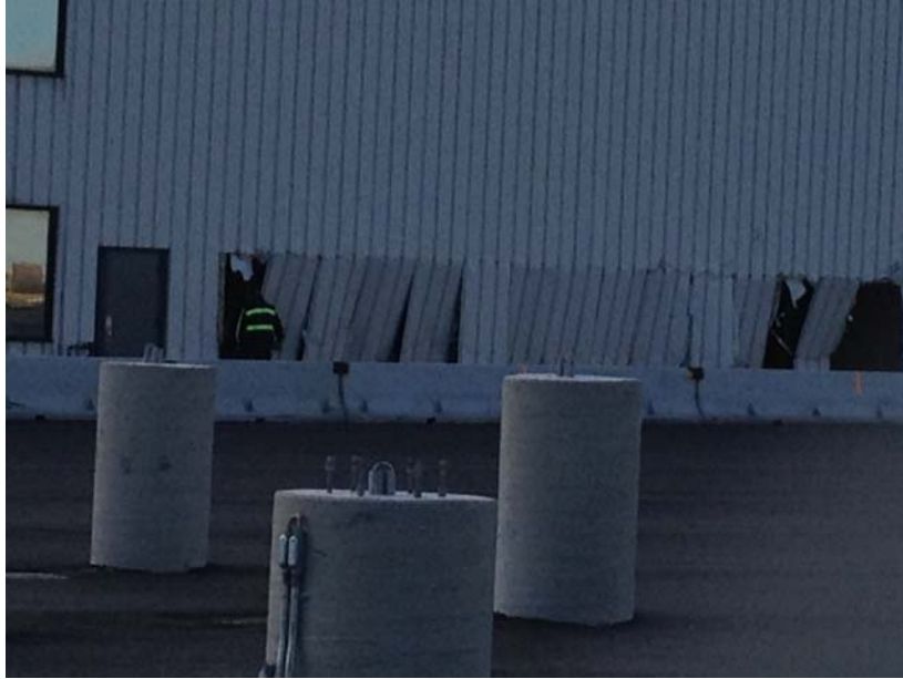
Figure 8: Wall damaged by waves and surge during Sandy
