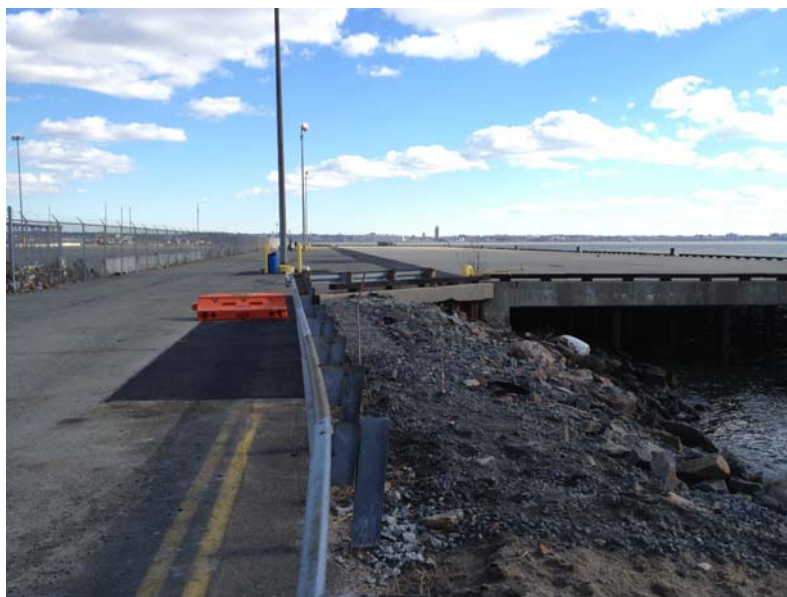
Figure 7: Revetment damaged during Sandy
