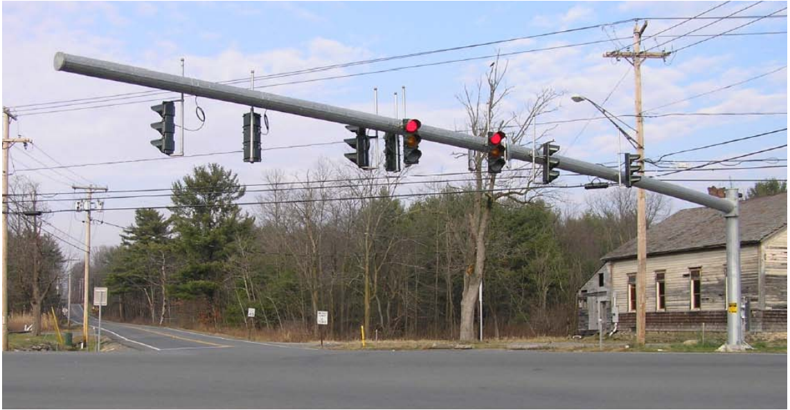
Figure 1.1: Cantilevered Mast-Arm Traffic Signal Structure [1]
