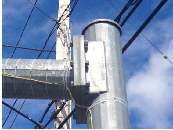
Figure 1.2: Mast-Arm Connection Detail
