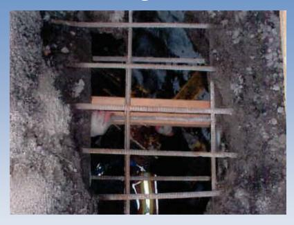
Collapse of closure pour in 2003 created hazardous conditions for motorists and required \$50,000 in emergency repairs.
