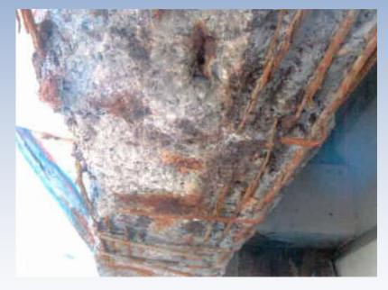
Rebar and tendons exposed and corroding due to deferred maintenance
