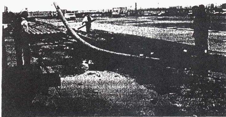
Fig. 2-4 Handling Fiber Reinforced Plastic Piling; Low Stiffness of some Composite Piling Materials.
