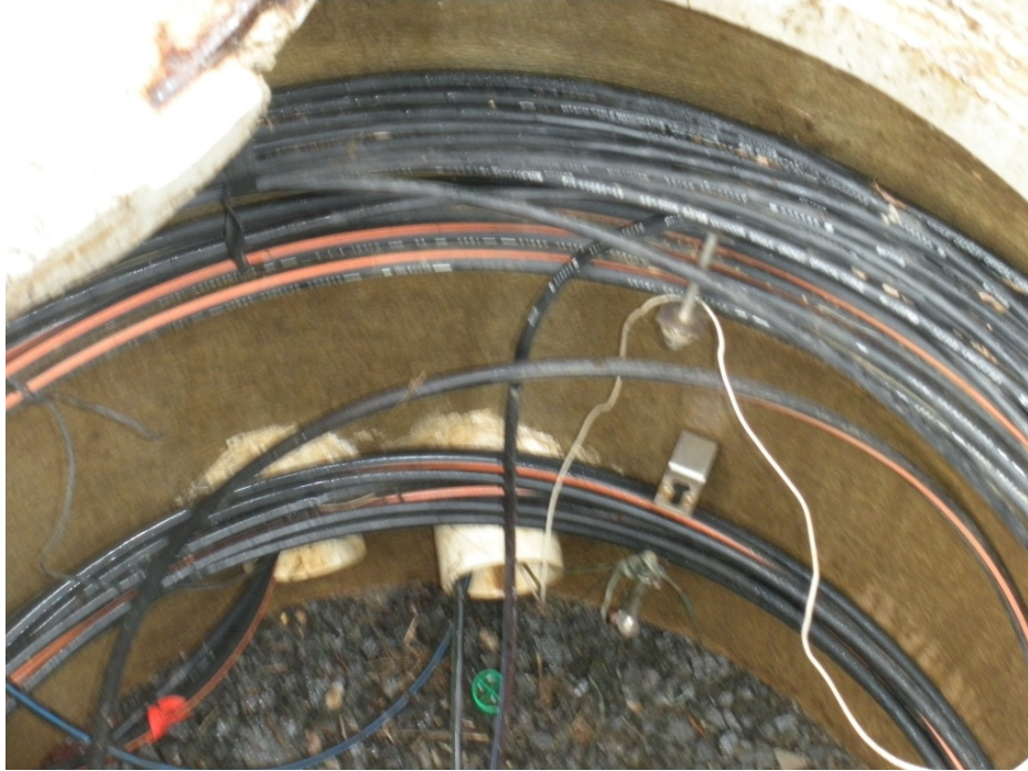
Figure 3: Closer view of conduits on one side. White wire entering one of the conduits is a trace wire. A small transmitter was connected to this wire to generate a signal that could be detected through the earth.
