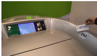
Figure 1-5. Save-As-You-Throw: Inlet Equipped with Magnetic Card-Reader (Source: Envac, 2012)
