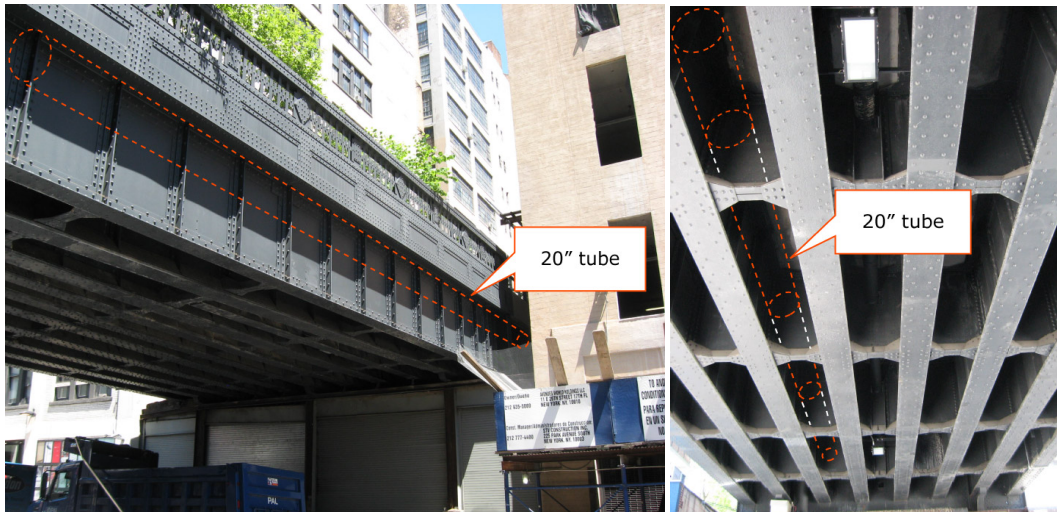
Figure 3-1. High Line, View From Street Showing Tube Location Along Side Or Between Girders
