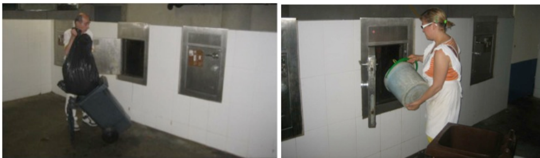
Figure 3-5. Central Waste Room (Pneumatic Collection of Refuse and Organics) at the Sta Caterina Market, Barcelona
