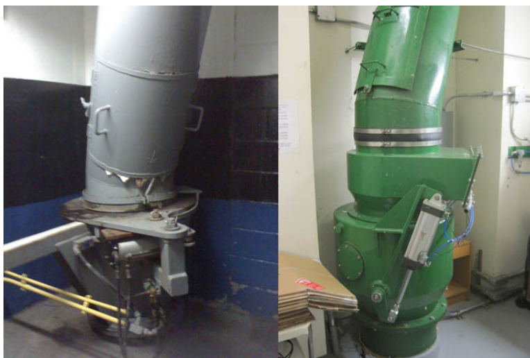
Figure 1-4. Base of RI Inlet Chutes, Diverter Valves 11 (Source: Ross, 2011)
