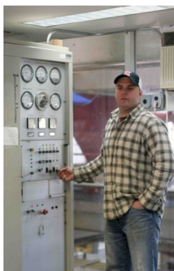
Figure 3-7. DSNY Stationary Engineers Turn on Exhaust Fans and Open Diverter Valves From Terminal Control Room (Source: Milford, 2010)
