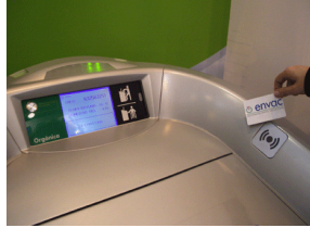
Figure 1-10. Inlet Equipped with Magnetic Card-Reader (Source: Envac, 2012)
