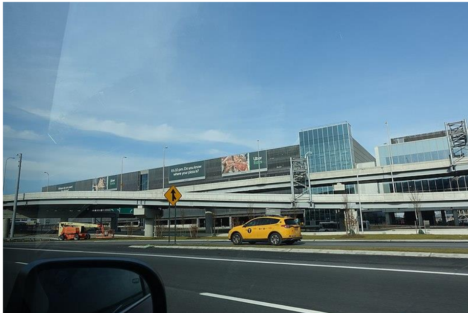
New Terminal B Parking Garage. Image Credit: Tdorante10, via wiki commons.wikimedia.org
