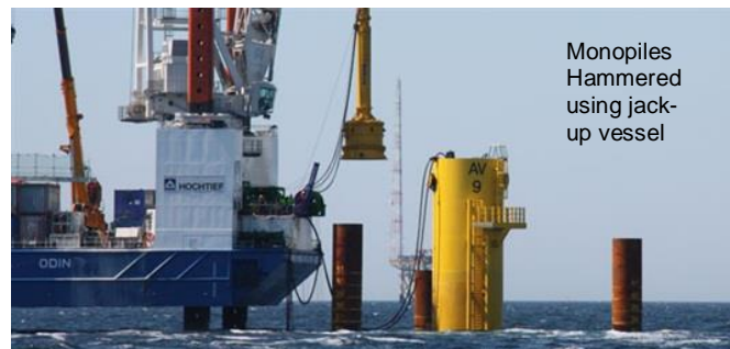
Figure 5. Offshore Wind Farm Installation Process
