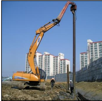
(a) Pile drilling
