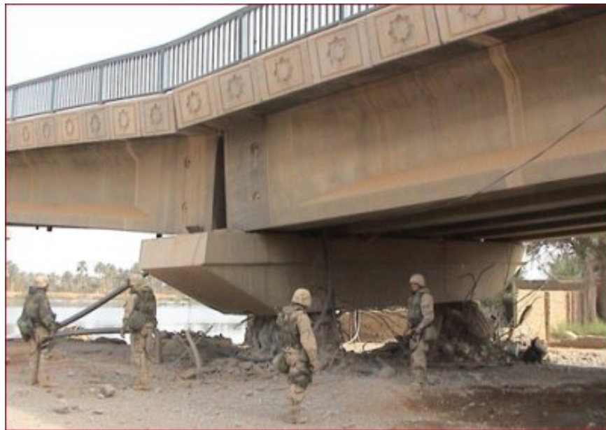
Figure 1.1 A bridge in Iraq damaged by a relatively small amount of explosives placed in a terrorist attack.
