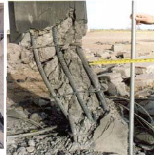
Bottom of Failed Column
