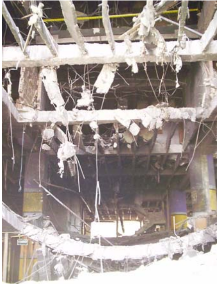
Figure 5.17: Damaged Club El Nogal Site. Undamaged column is pointed by an arrow.
