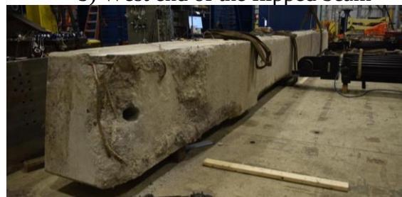
c) East end of the flipped beam
