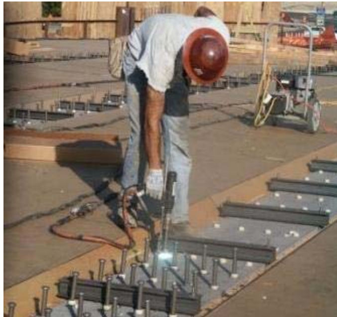
Figure 4. Use of portable semi-automatic welding machines to install headed shear connectors on girder flange. (Stud Welding Product, Inc.)
