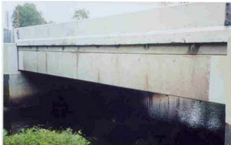
Figure 1. Corrosion due to transverse deck cracks in a bridge in New Jersey. (Saadeghvaziri and Hadidi, 2002)
