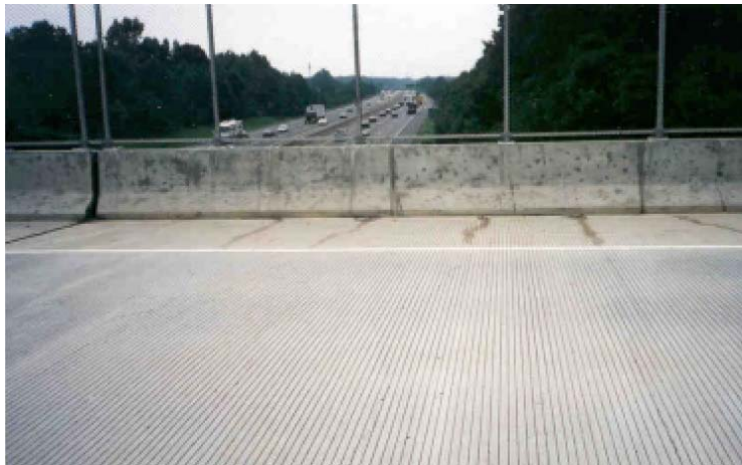
Figure 2. Transverse deck cracks on a bridge deck in New Jersey. (Saadeghvaziri and Hadidi, 2002)
