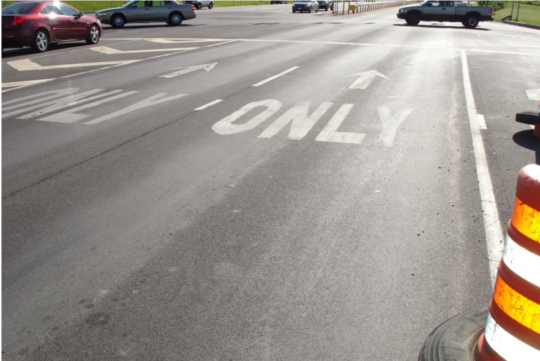
Figure 7 – Flushing at Intersection on Rt 5
