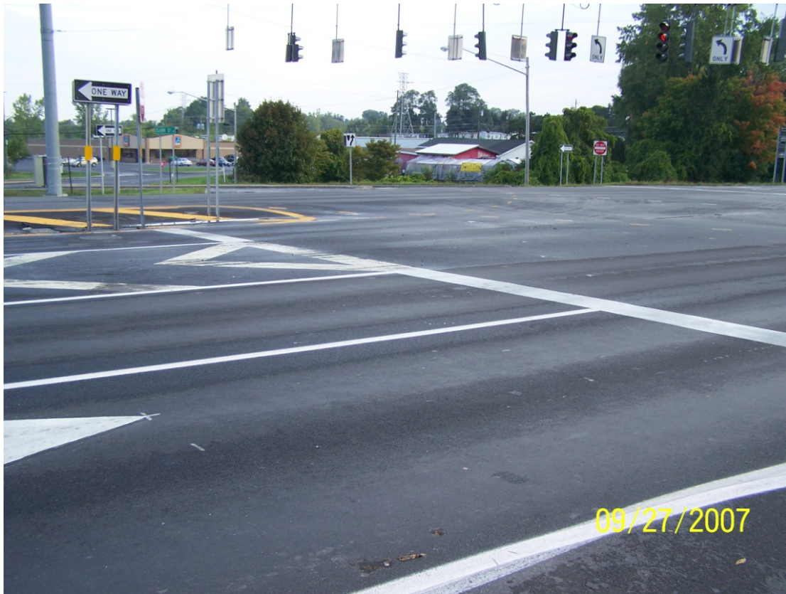
Figure 4 - Flushing at Intersection of Rt 5 (< 30 Million ESAL's)
