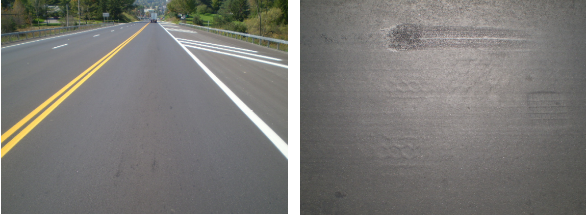
Figure 6 – Flushing Located on Rt 20 in Morrisville, NY
