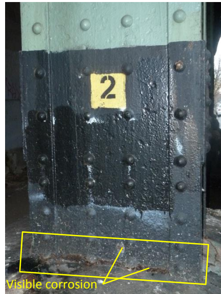
Figure 4. Bridge column typical conditions at base
