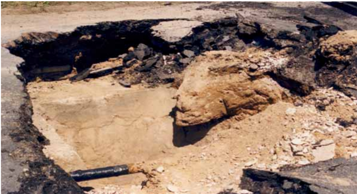
Figure 1.4 (a). Collapsed northwest approach of the Peckman's River Bridge roadway showing utility pipe.
