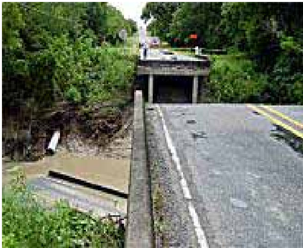
Figure 1.2. Recent Scour Failure of a Ovilla Road Bridge in Ellis County, TX.
