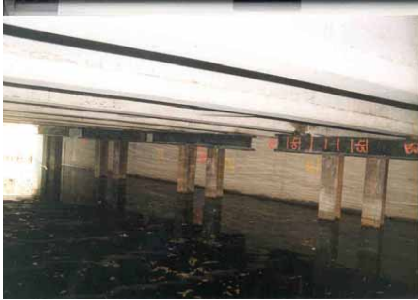
Figure 13.15. Exposed Pile Bents at Peckman's River Bridge on Route 46.
