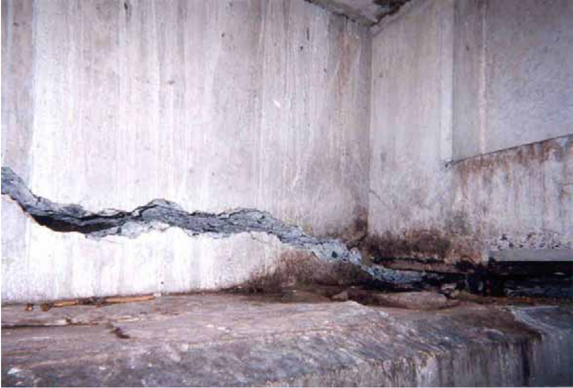
Figure 1.3 (b). Abutment Settlement at Peckman's River Bridge.
