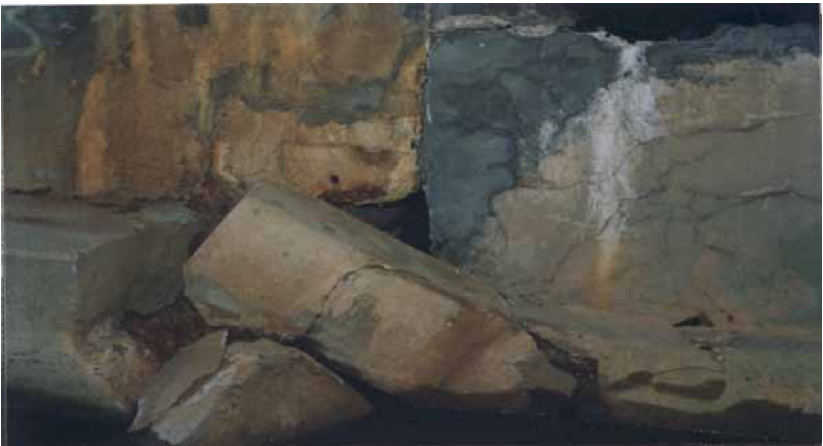
Figure 1.4 (c). Collapsed original north abutment built in 1890 founded on Spread footings on soil and undamaged widened abutment founded on piles, constructed in 1925.
