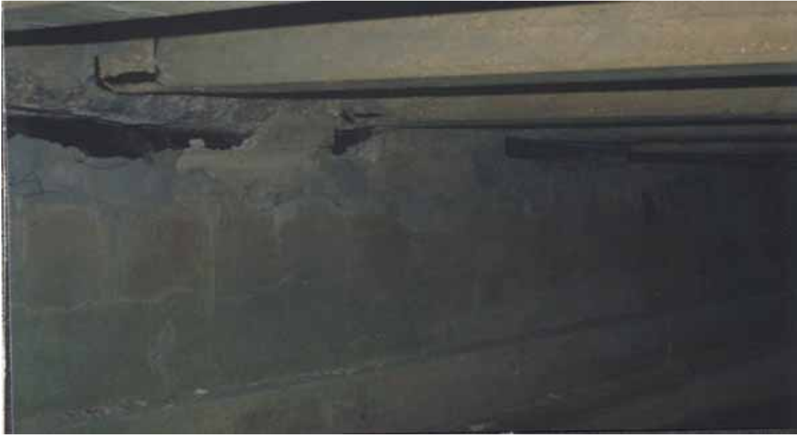
Figure 1.4 (d). Settlement of the north abutment of the Peckman's River Bridge (severe damage at the section not founded on pile).
