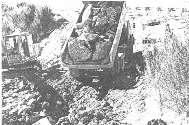
Figure 6.12. End-dumping of riprap (Smart, 1990).
