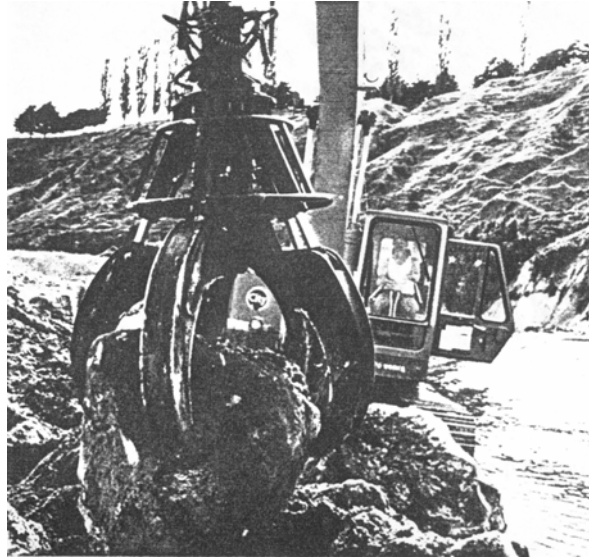
Figure 6.13. Riprap placement by grab (Smart, 1990).
