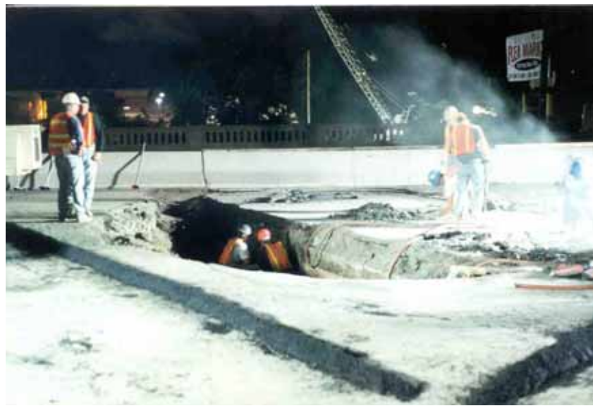
Figure 1.3. Failure of Approach at Peckman's River Bridge after Hurricane Floyd Struck.
