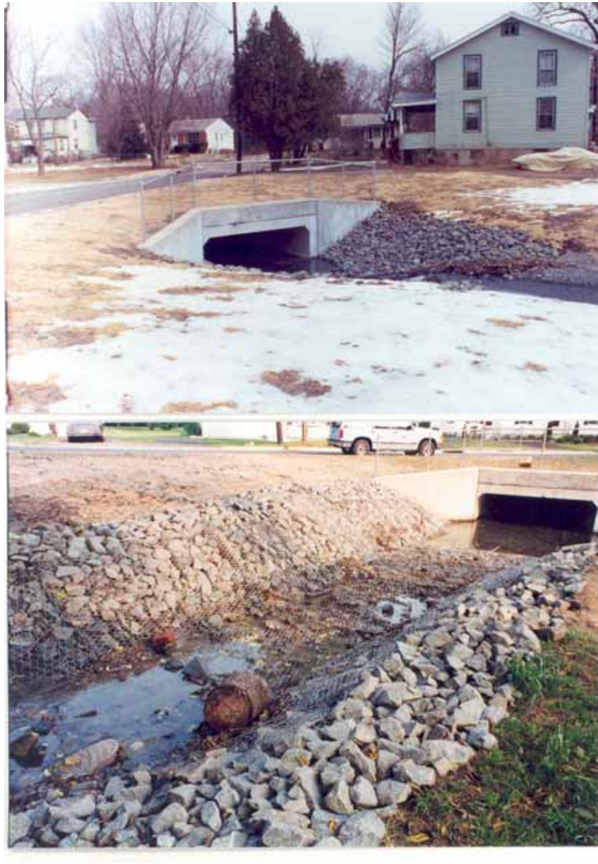
Figure 7.2. Use of Wire enclosed Riprap at Burlington County Bridge No. 128a.
