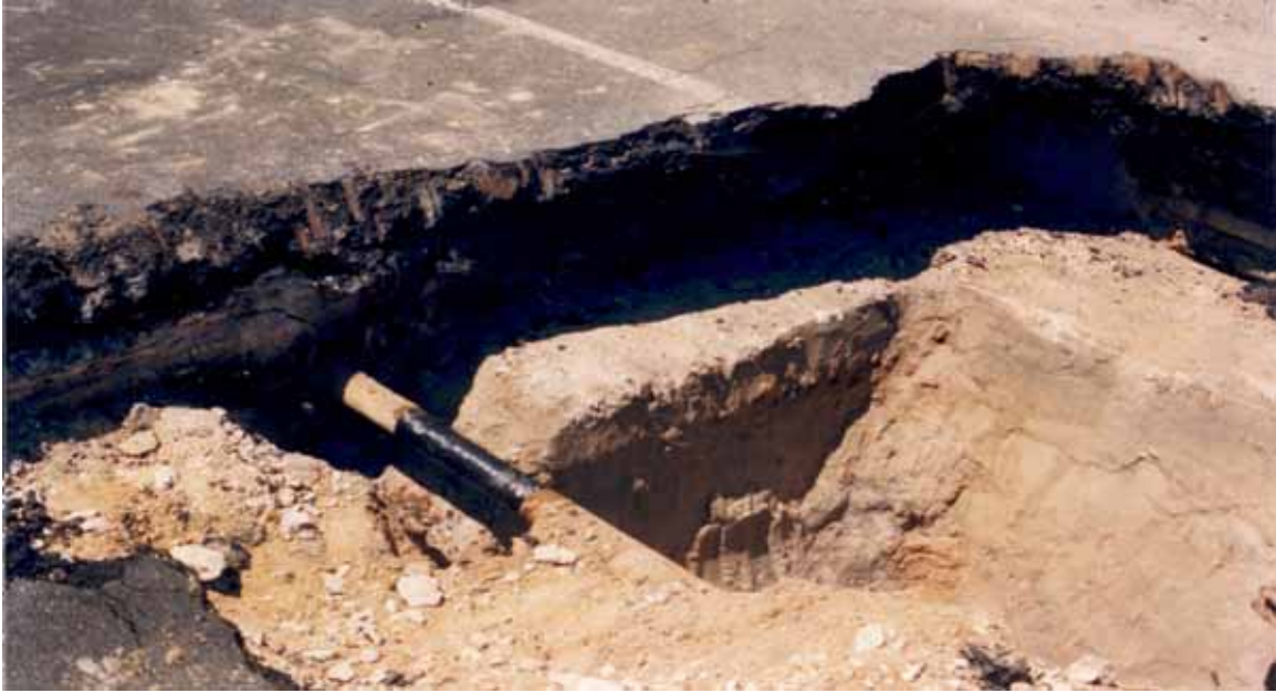
Figure 1.4 (b). Collapsed northwest approach roadway of the Peckman's River Bridge.
