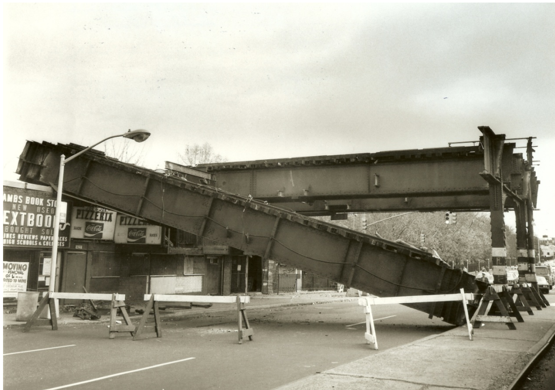
Photo 1: Demolition of the Third Avenue El
