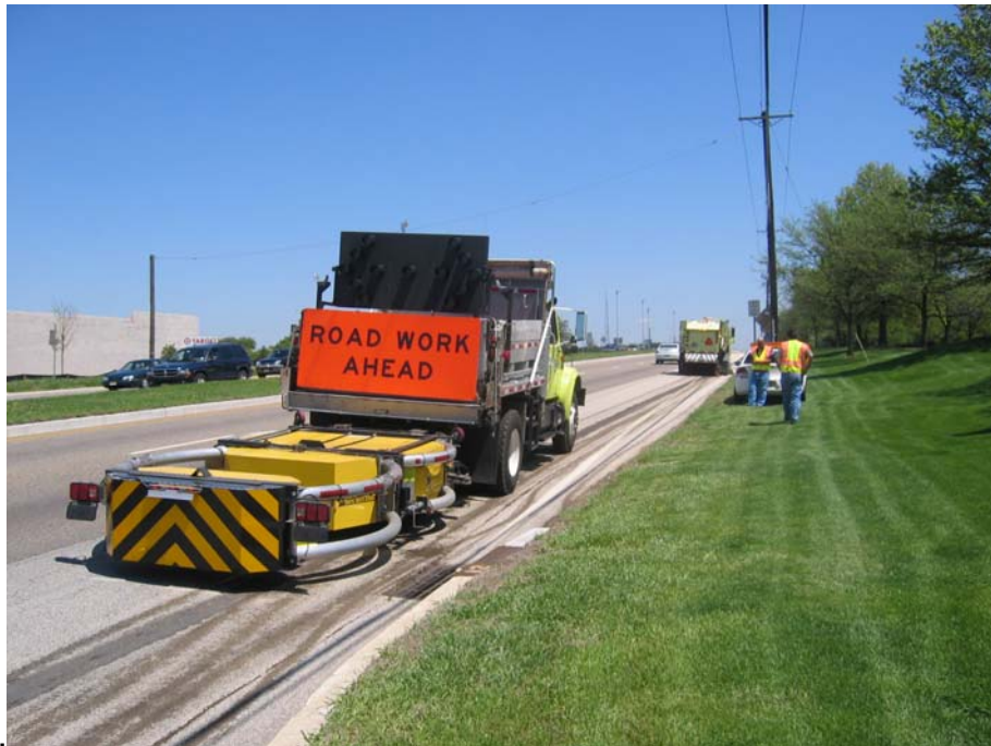
Figure 2. NJ Route 38 Eastbound Right Shoulder Sweeping Operation in Mount Laurel
