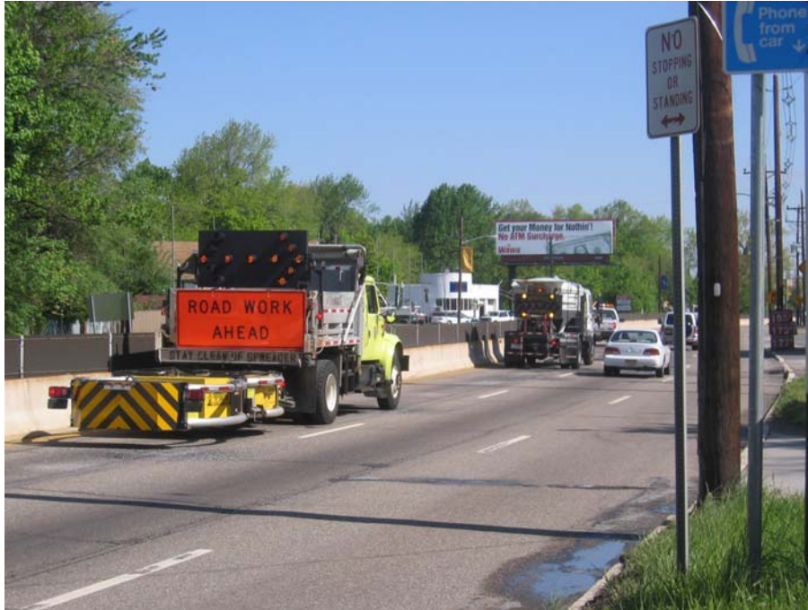
Figure 1. U.S. Route 130 Northbound Haddon Township Pothole Patching Operation.
