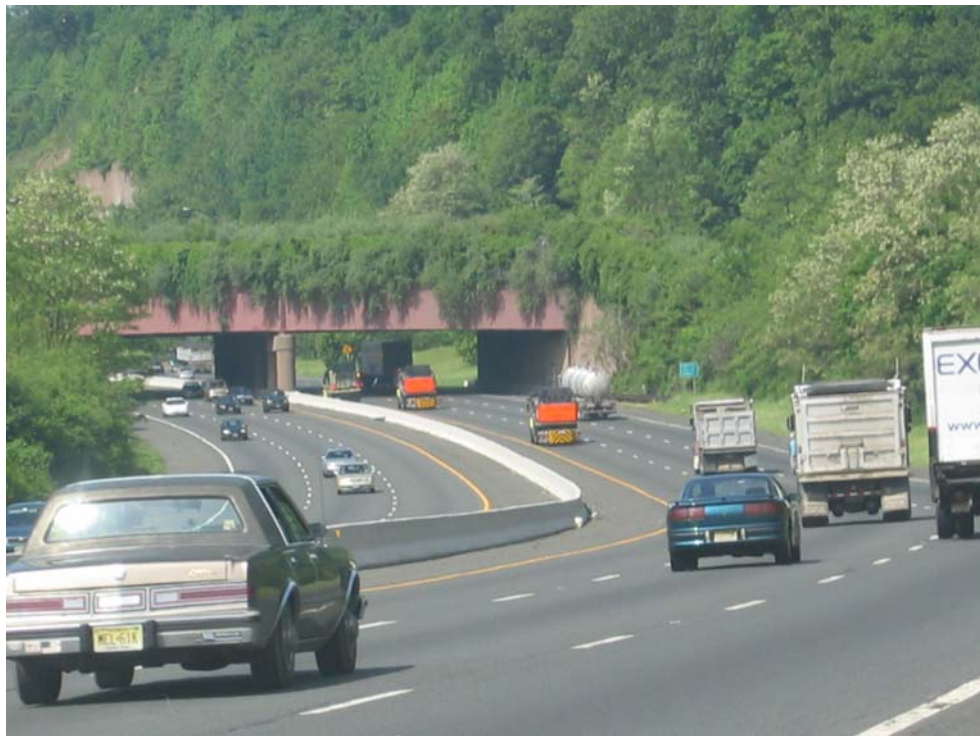
Figure 4. Landscape spraying operation on Route I-78, on the inside shoulder.
