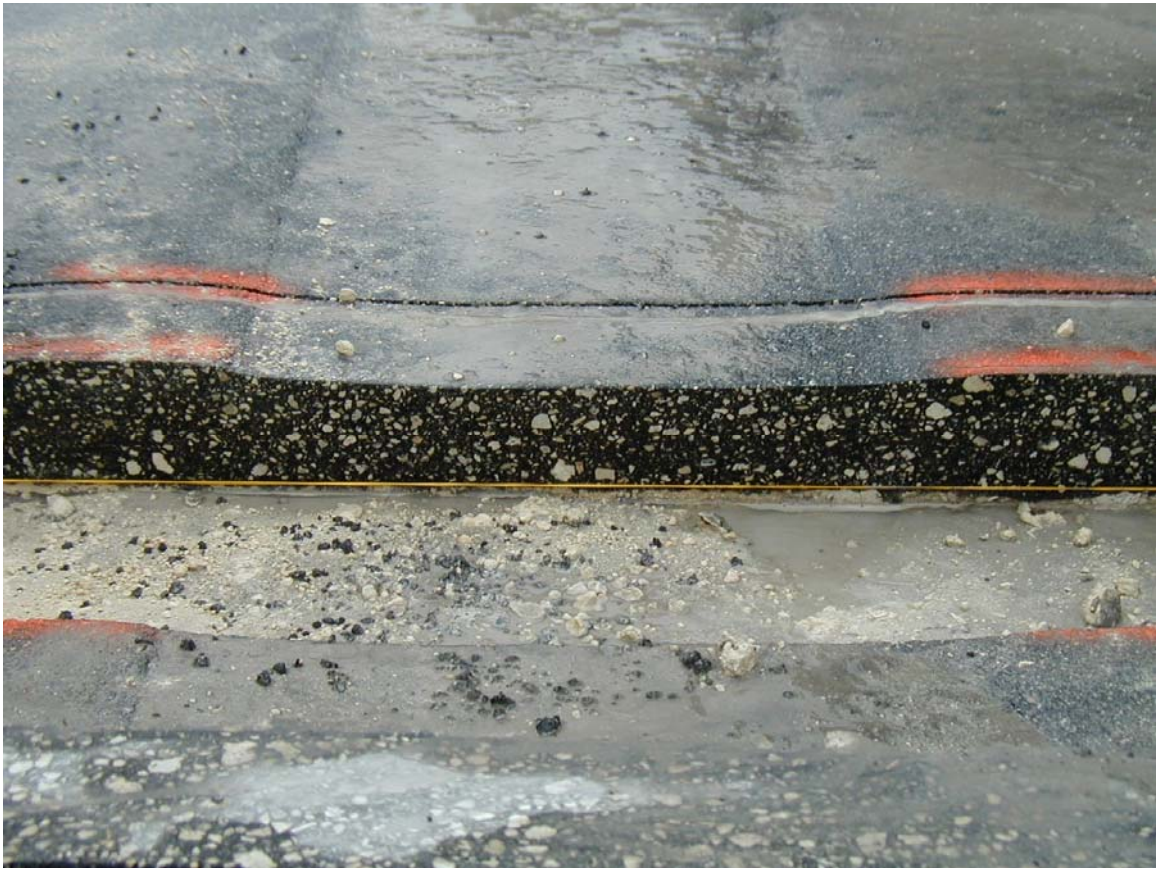
Figure B-3 Section 1-B showing no deformation of the base layer – Most of the deformation is due to asphalt compaction
